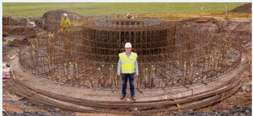
Wind turbine groundworks, Stewart Energy
